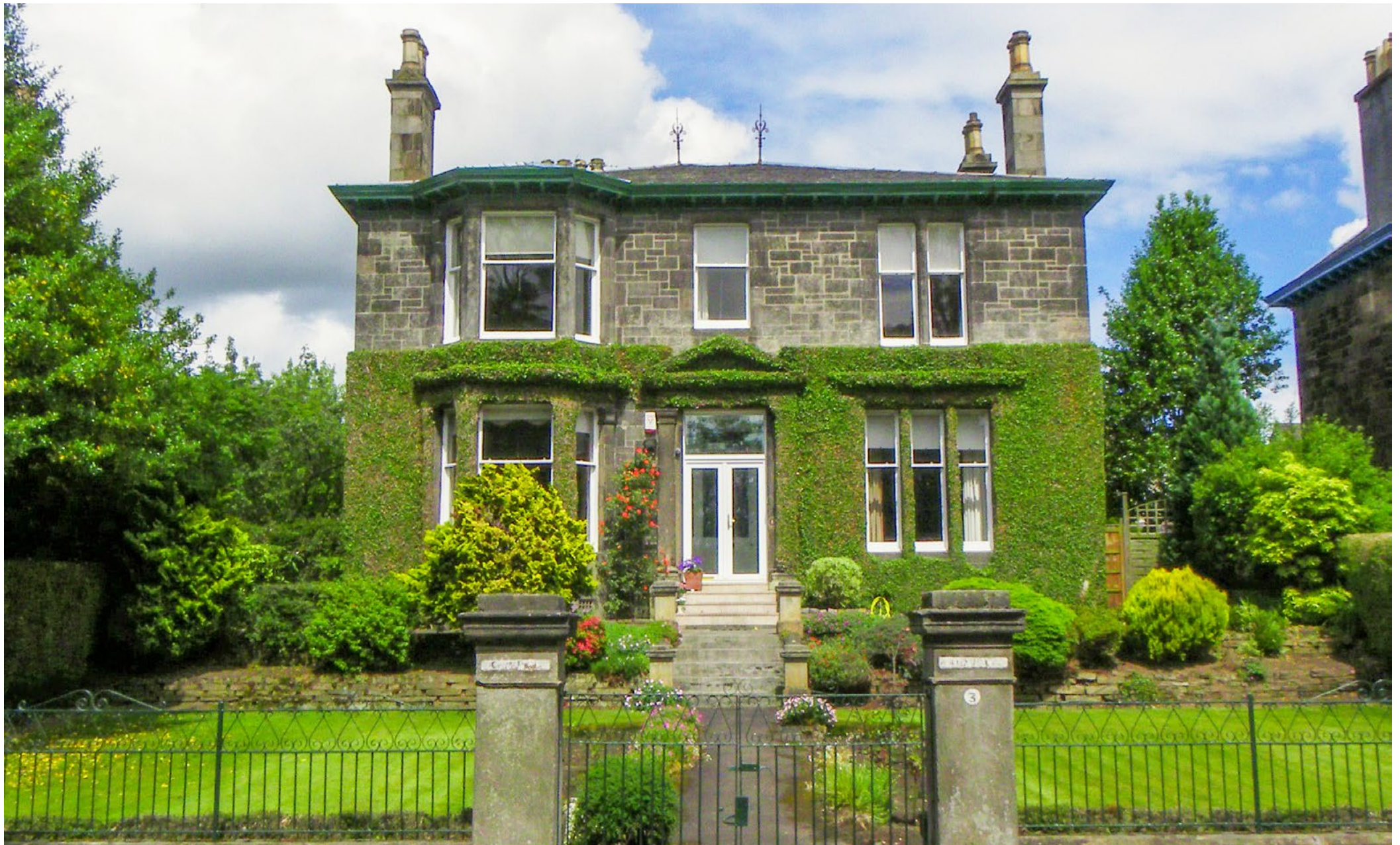
Clare House, 3 Bowling Green Road, Mount Vernon
